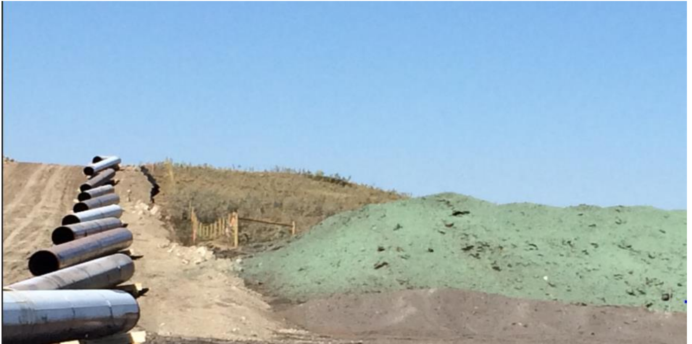
HDD pipe on the hill East side Chapleau lake & the soil stabilization (tackifier) 622+224
