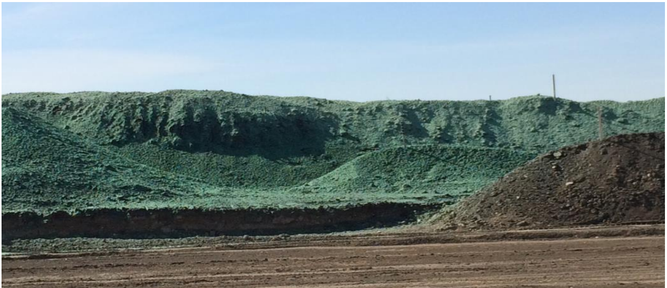
HDD pipe on the hill East side Chapleau lake & the soil stabilization (tackifier) 622+224
